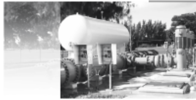
The color purple is used to identify pumps, tanks and pipes carrying reclaimed water for reuse. The photo above and on the cover shows a reuse facility in Pompano Beach.
